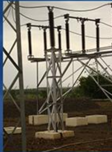
33KV Substation work
