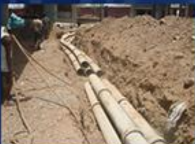
CWC -Underground HT cable laying
