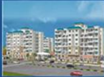
Residential + Commercial electrification including of HT work.
