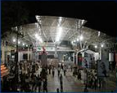
C. Railway - Street Light & Platform electrification of Main entrance.
