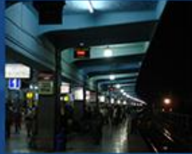
C.Railway Pune - Total lighting improment of Platform No. 1,2,3 & 4 at Pune station
