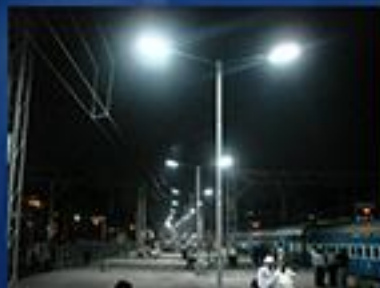
C.Railway - Street Light work
