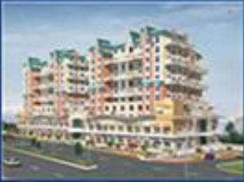
G.M.Kenjale - Light house - Com.& Resid. electr. work with of 22KV indoor substation work.
